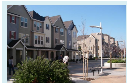
Buildings should be oriented to activate pedestrian plazas or other public spaces.
