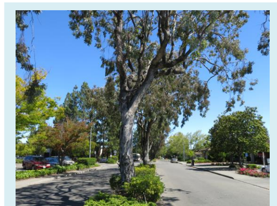
Attached sidewalk condition on Enterprise Drive
