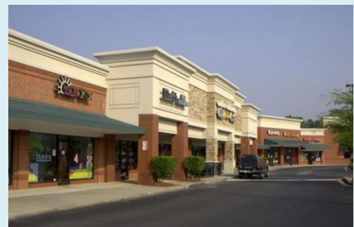
This façade renovation incorporates covered walkways and features façade articulation.
