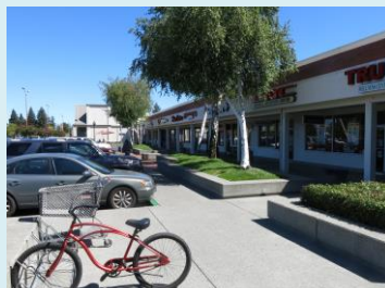
The Central Commercial subarea is a cluster of centers providing retail and services to the community.
