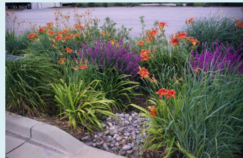
Incorporate LID features, such as bioswales, into parking lots, to slow stormwater run-off.
