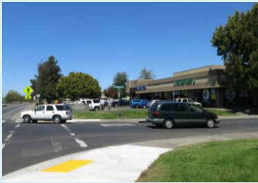
The Triangle Business subarea is a mixed-use employment center with freeway presence near the SMART rail line.
