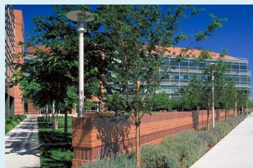
Buildings should be designed to provide an attractive appearance along public rights-of-way.
