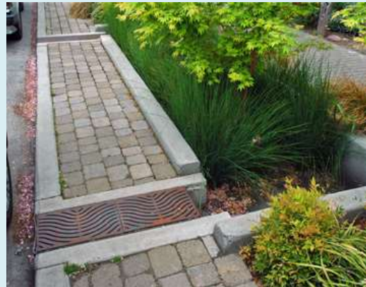
Example of a green gutter.
