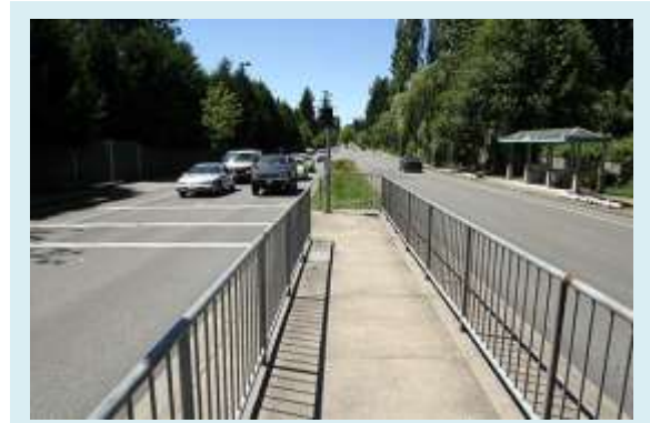
As an alternative, an L-crossing may be considered for the midblock crossing on RPX.
