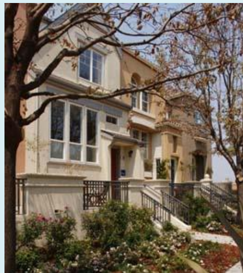
Provide a diversity of housing types and styles with shared common space.
