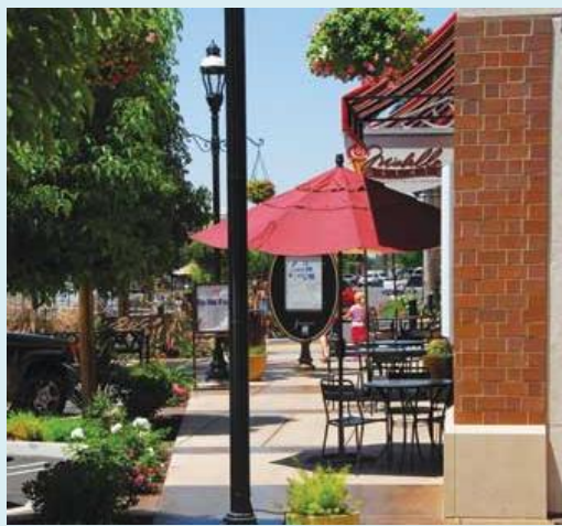
Accent colors or materials should be used to highlight architectural building features.
