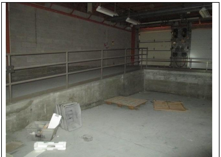
6. View of the former shipping & receiving area.
