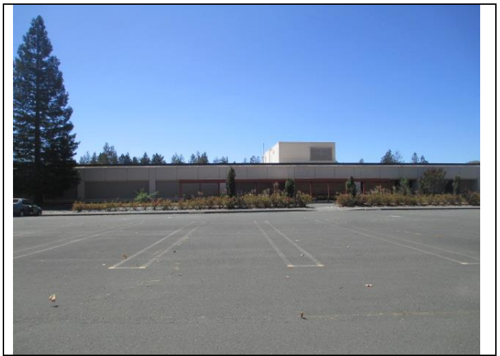
2. View of the east side of the building.
