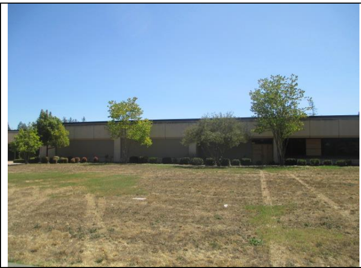
1. View of the north side of the subject property building.
