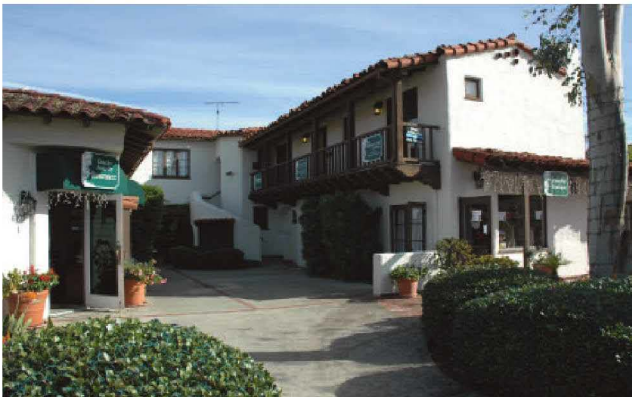
An Apartment House with commercial uses.
