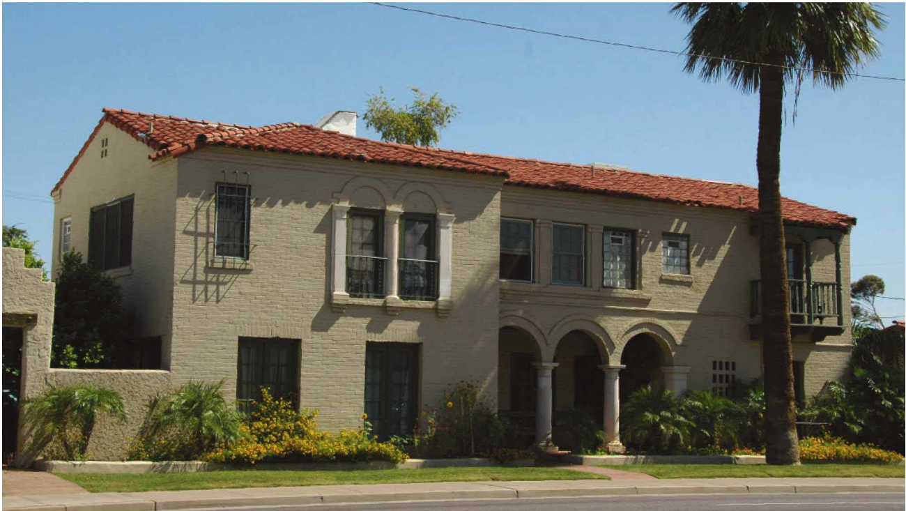
A Mansion Apartment, scaled to a medium-density neighborhood, with all units accessed from a central entry
