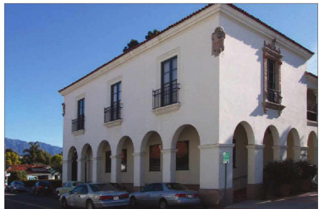
An example of an arcade encroaching the public ROW. The arcade provides the only means of circulation along the ROW.
