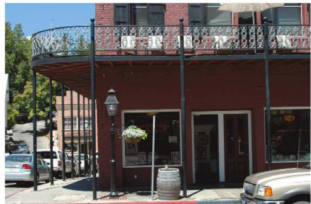
A two story gallery where the second floor is uncovered.
