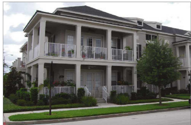
Example of wrap-around projecting porch on the front and side street facades
