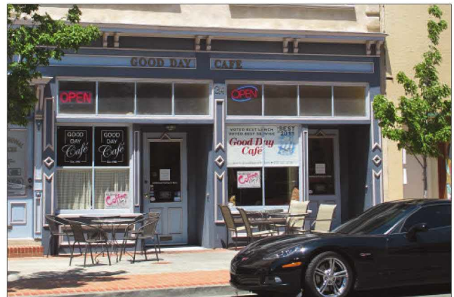
Example of a shopfront with a recessed entrance.
