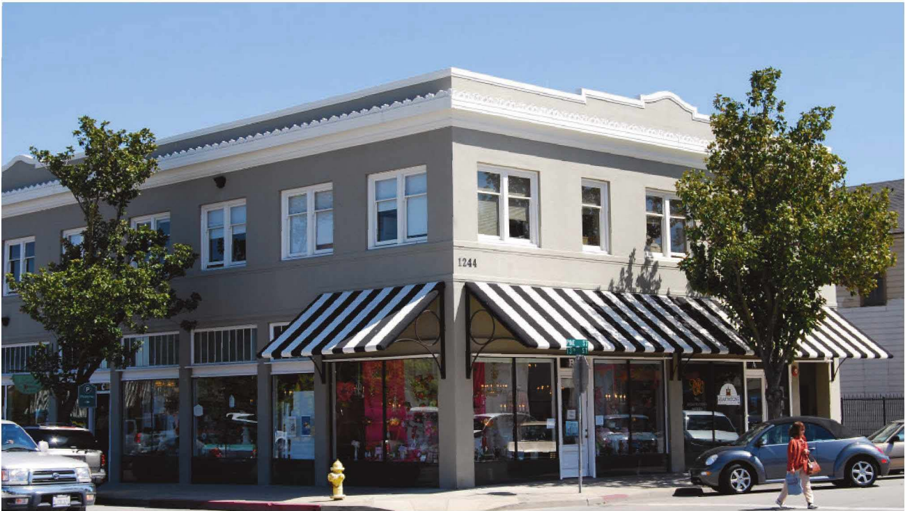
A two story Main Street building with shopfront frontage with awnings
