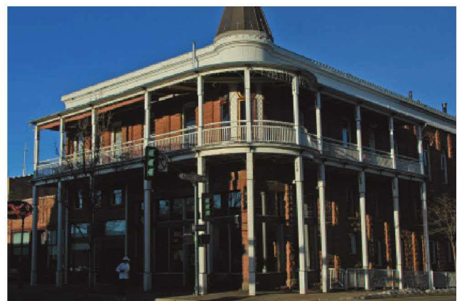
A two-story gallery frontage.
