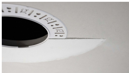
Partially finished mud ring, showing cross-section detail.
